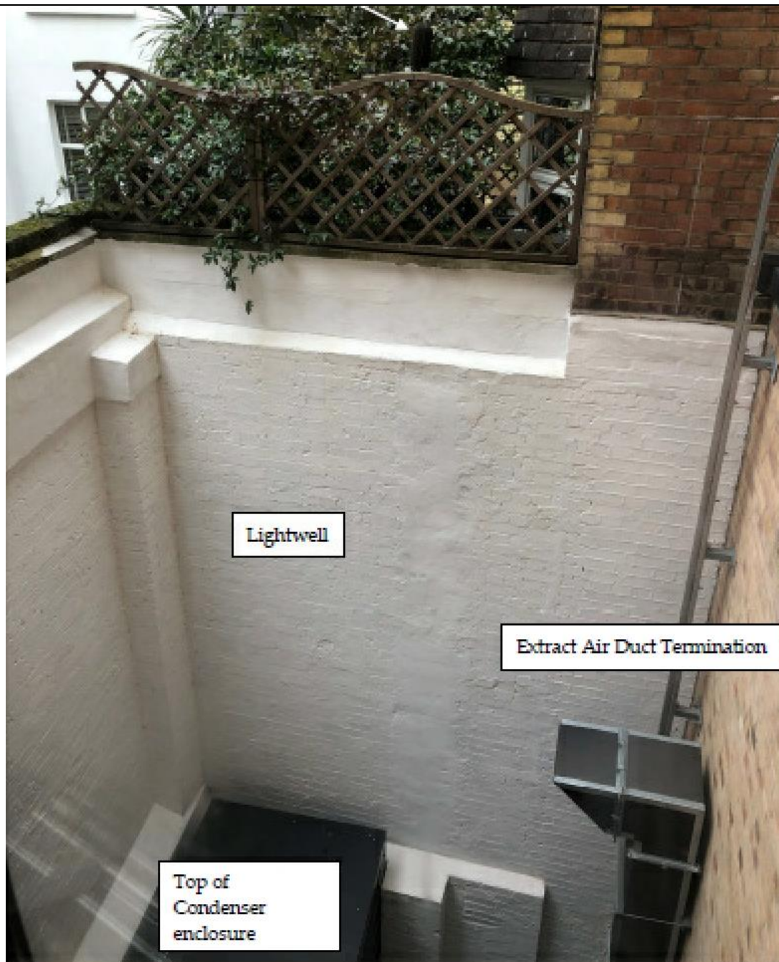
External sunken lightwell to rear
