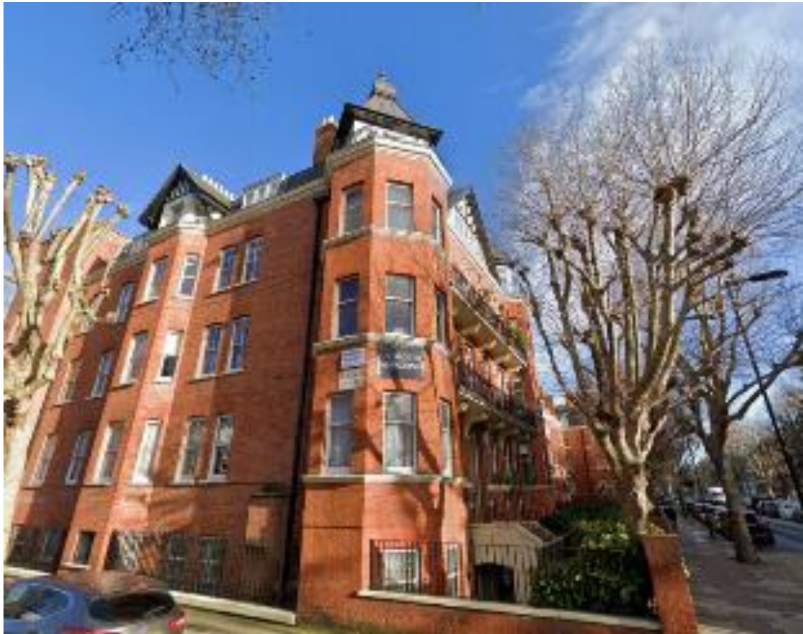
Front Elevation; Flat 44 is at 2 nd Floor with the windows on the corner.
