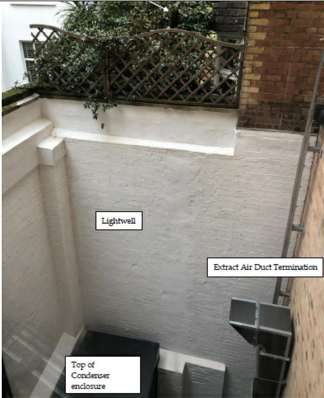
External sunken lightwell to rear
